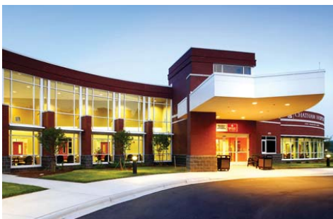
Chatham Hospital, Siler City, NC
